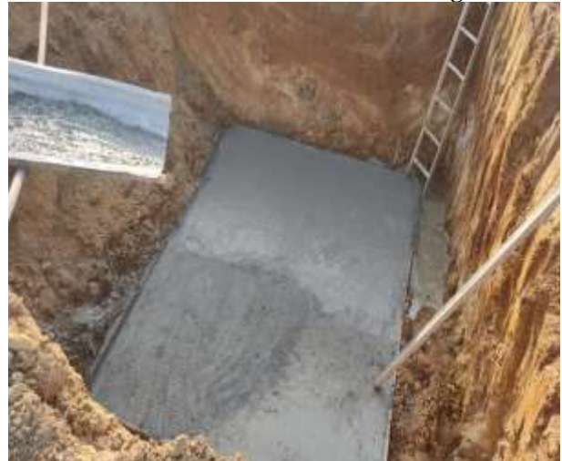
PCC Concrete Work
