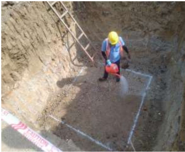
Anti Termite Work
