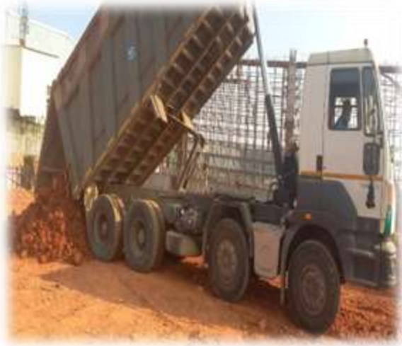
Soil Filling and Compaction
