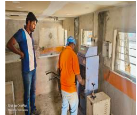
PCC Concrete Trial Mix Testing
