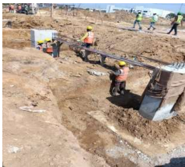
Plinth Beam Shuttering and Concrete Casting
