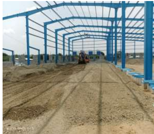
GSB Levelling and Compaction
