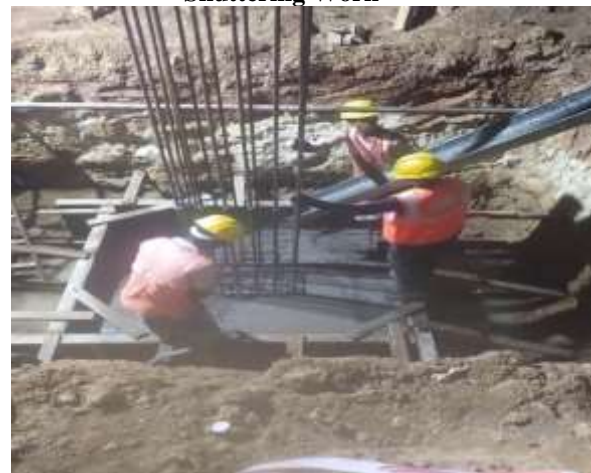
Footing Concrete Work, Pedestal Barbending & Shuttering
