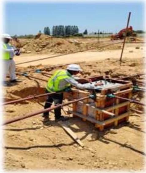
Anchor Bolt Fixing & Checking
