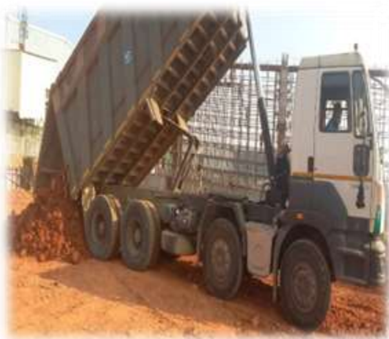
Soil Filling and Compaction
