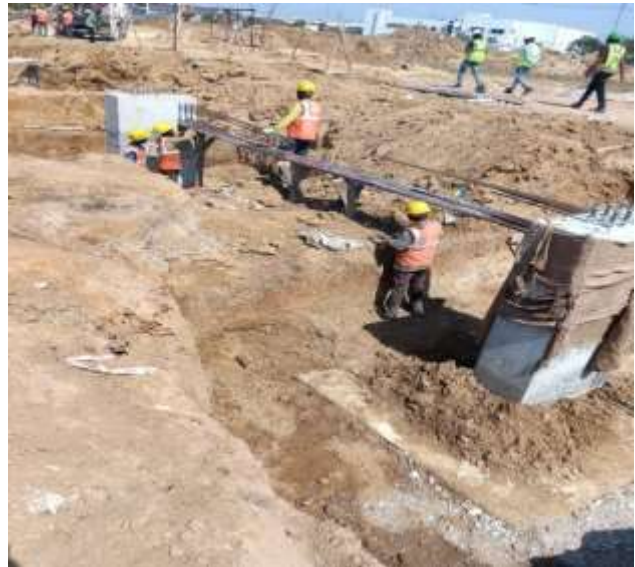
Plinth Beam Shuttering and Concrete Casting
