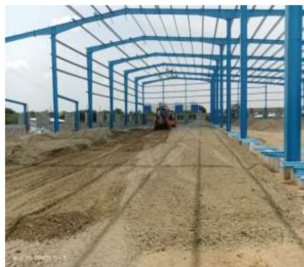
GSB Levelling and Compaction
