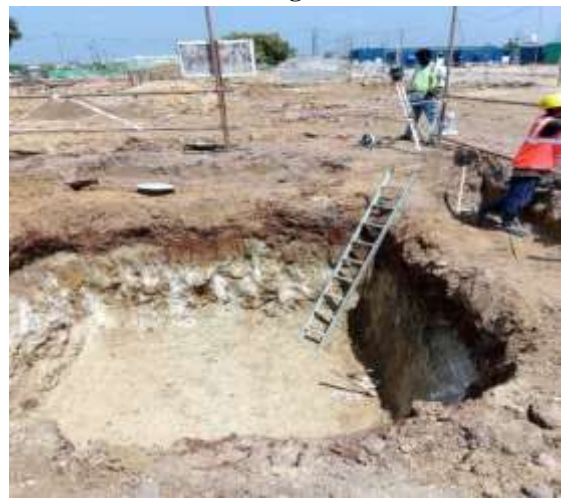
Footing Levelling and PCC Marking Work
